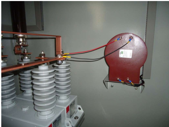
C.T. for unbalance protection
