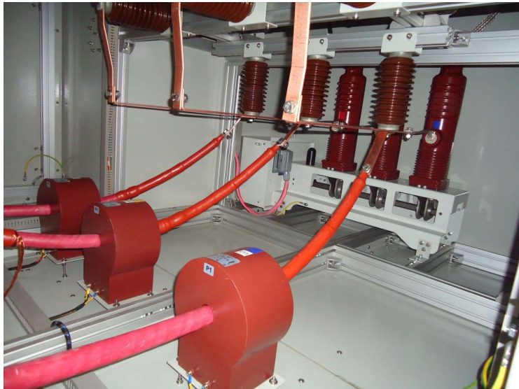
Vacuum circuit breaker at the entry
