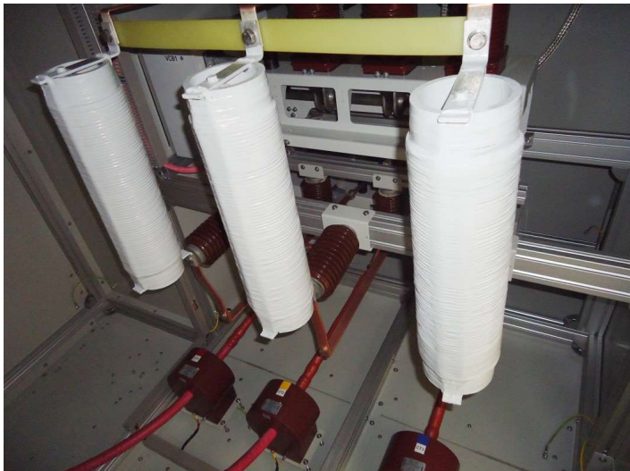
Equipped with inrush reactor
