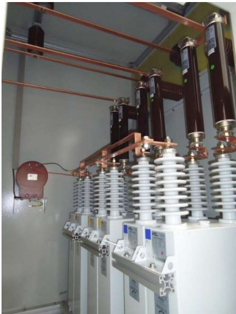
Capacitor protection fuses
